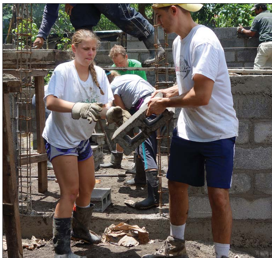
The team helped build two houses in just four days.
